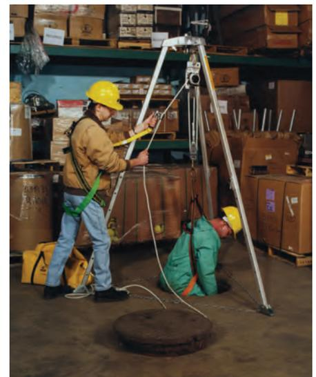
A secondary fall arrest system is recommended
